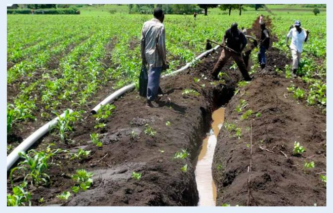
LAYING THE PIPES DOWN IN SANZARA FOR THE GRAVITY FLOW SCHEME, BRINGING WATER FROM THE RIVER TO IRRIGATE FIELDS AND PROVIDE STEADY WATER SUPPLY TO THE COMMUNITY. © IUCN Uganda
